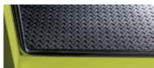
Container floor with crosshatch metal pattern surface
